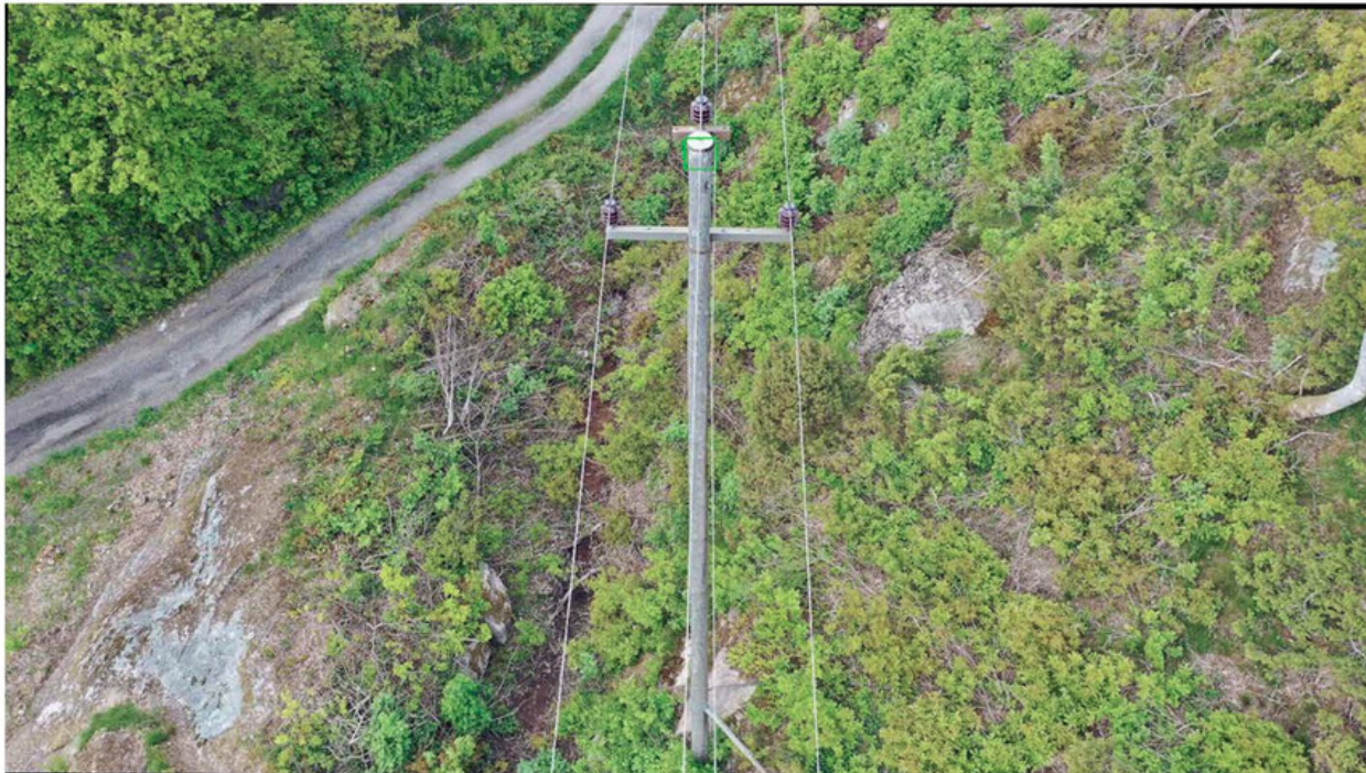
Pole defects scanning approach
